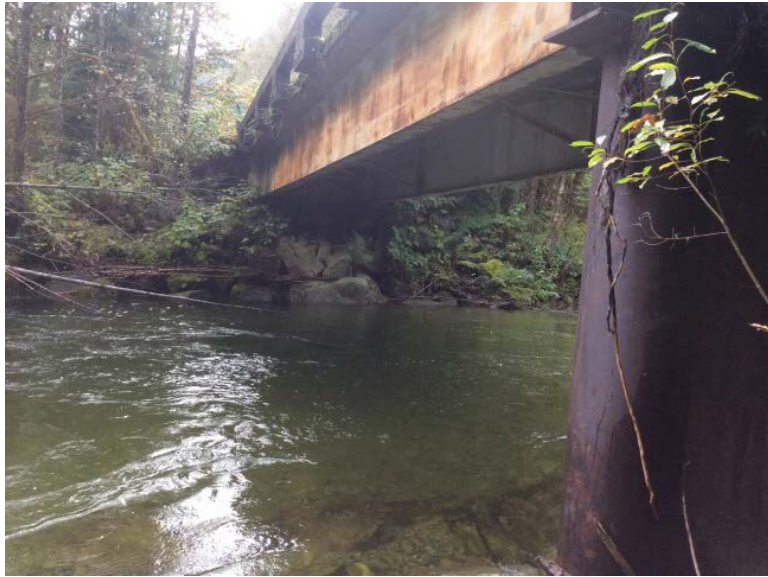
Left Bank Abutment when facing downstream
