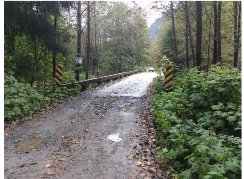
Approach from Right Bank when facing downstream
