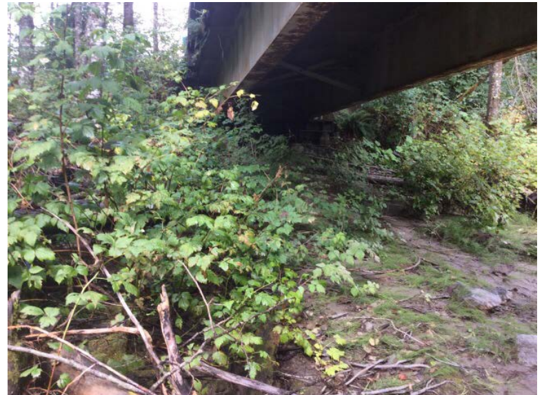
Right Bank Abutment when facing downstream
