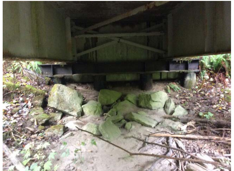
Right Bank Abutment when facing downstream
